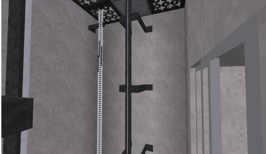
Install magnets above the top of the door at each landing. Brackets are available for supporting the ends of the tape.
